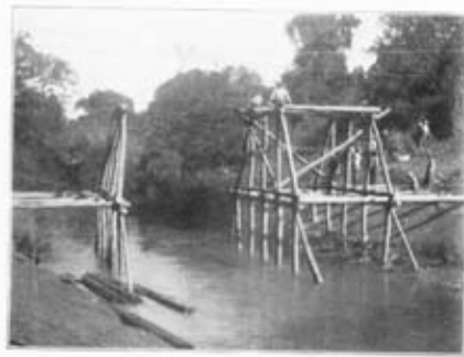
3. Timber Trestle Bridge, length 140 ft., centre span 20 ft.
