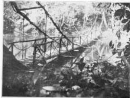
4. Suspension Foot-Bridge made with Bamboos and Creepers, 60 ft. span.
