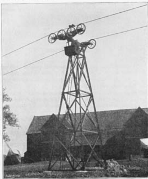
PHOTO 3.—Type of Iron Trestle and Bearing Pulleys.
