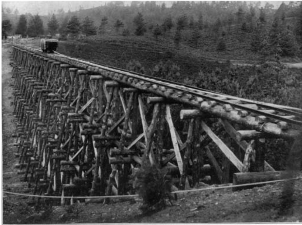
3. Trestle Bridge to carry 3' 6" Railway. Span 334 feet; maximum height 40 feet.
