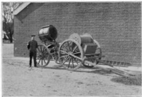
24 inch Projector on Trail Carriage, with concentric cable on converted gum timber.
