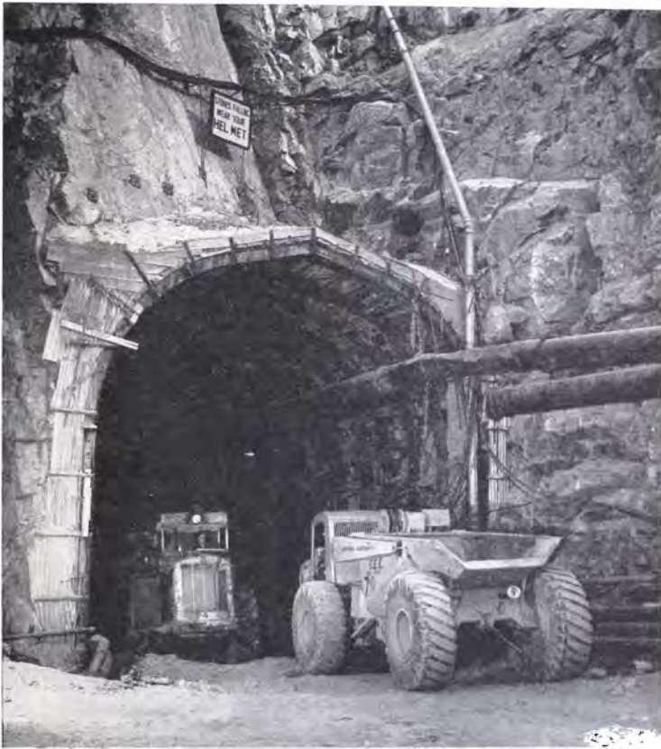
Photo 5. —T 1 Power Station—Tournarockers in the access tunnel.
