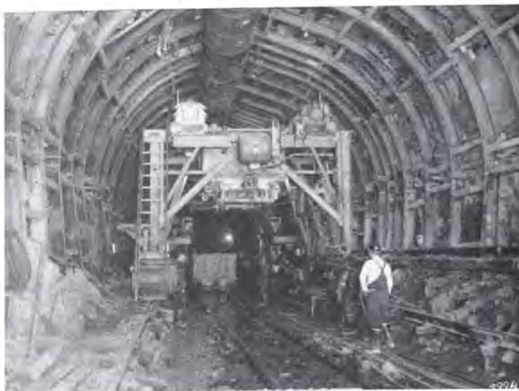
Photo 3. —Eucumbene-Tumut tunnel, "Cherry-picker" in operation.
