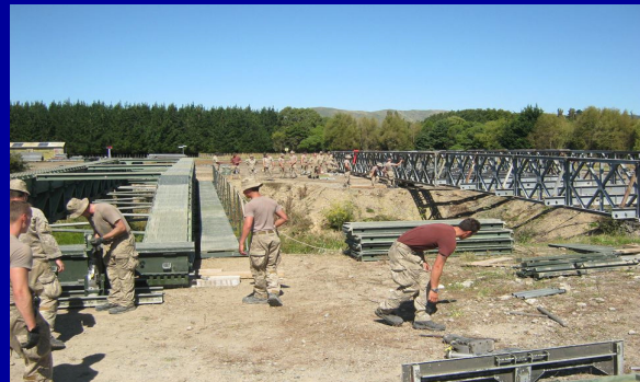
The Medium Girder Bridge (MGB) on the left, and the Extra Wide Bailey Bridge (EWBB) on the right are two forms of kitset bridging employed by RNZE.
