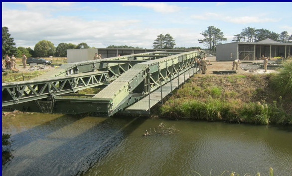
The MGB with launching nose allows a bridge to be constructed and launched across an otherwise impassable gap.
