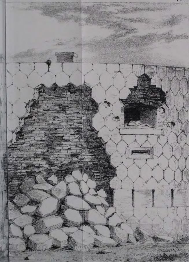
D, SHEWING ITS CONSTRUCTION & THE EFFECT OF A CHARGE OF 64 LBS.
